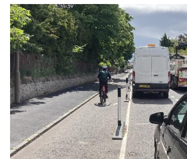
Figure 6.1: With-flow light segregated cycleway example
